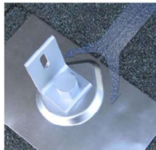
Flashing designed to redirect water flow.
