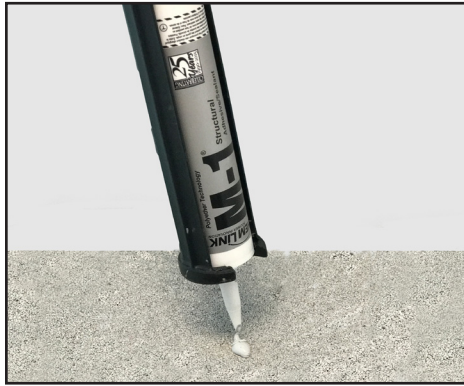
STEP 2: Apply a generous amount of roof sealant into pilot hole.
