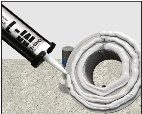
STEP 7: Apply M-1 Sealant to E-Curb, per ChemLink guidelines.
