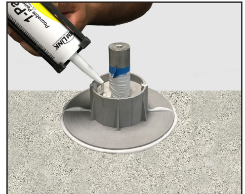
STEP 9: Fill E-Curb with 1-Part filler and remove tape.
