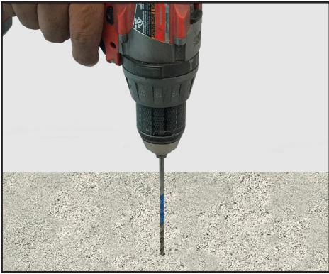
STEP 1: Use carbide bit to drill pilot hole (1/4" diameter pilot hole for 3/8" fastener.)
