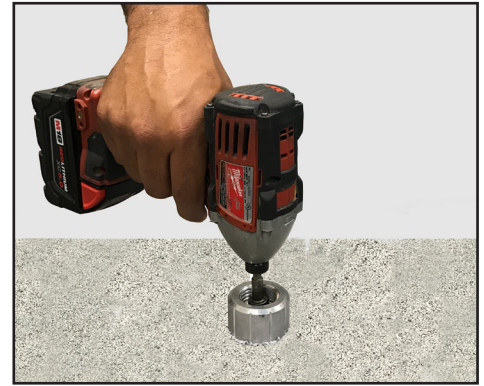
STEP 3: Using a cordless impact wrench, fasten lag bolt to rafter through base until seated.
