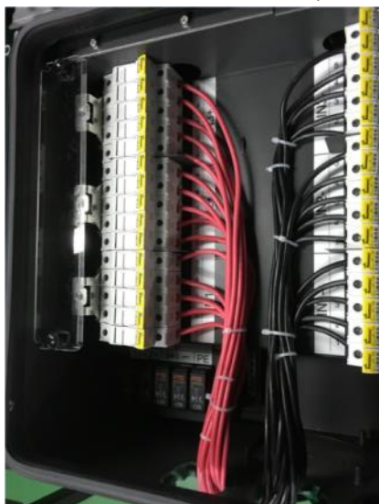
Figure 2.27- DC Input Cable Connection (standard wiring box)
