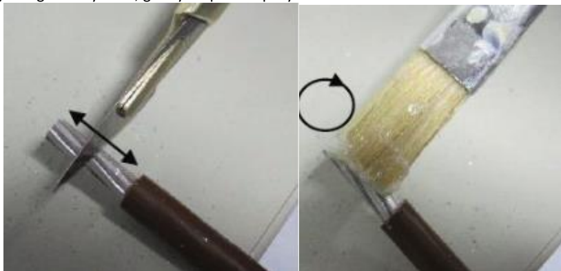
Figure 2-38 Preparing aluminum wires prior to connecting
