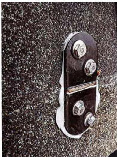
**Figure 4b.** Mount failure mode.
