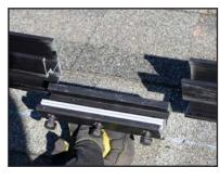
The rail splice is inserted into the channel where two rails but together. Three bolts are used to tighten the splice.
