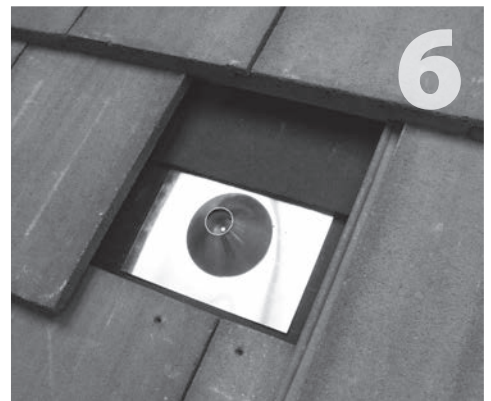
Take care to do a quality installation. When using the paper method, cut a piece of paper 18" wide to slide under the course above, and over the primary flashing of the mount.
