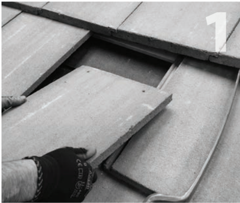
Remove tile at selected location of mount.
