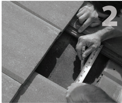
Locate and mark center of rafter.
