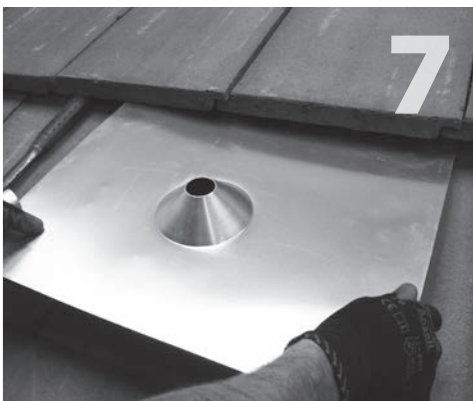
Cut a hole in the tile removed, with room to get the post through. Replace tile in position. Insert post and tighten into place. Install the 18"x 18" flashing and apply sealant around the opening.
