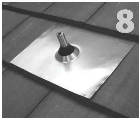
Apply sealant where post and flashing meet, and install counter flashing collar. (Be sure to seal off the post from weather exposure with the sealing washer (item 8), in the interim before racks are installed.)
