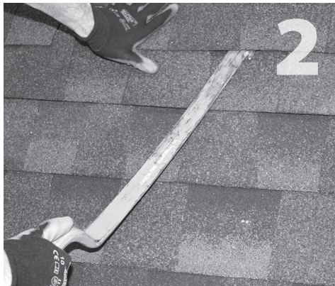
2 Carefully lift composition roof shingle with roofing bar, just above placement of mount. Remove nails as required. See "Proper Flashing Placement" on next page.
