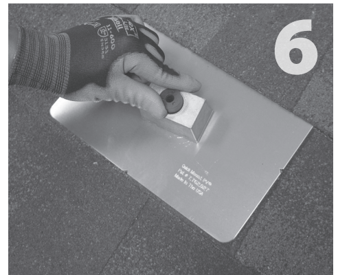
6 Slide the flashing into position. Insert the rubber plug into the QBlock cavity.
