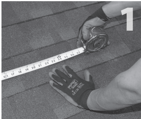
1 Locate, choose, and mark centers of rafters to be mounted. Select the courses of shingles where mounts will be placed.
