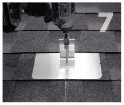
Prepare lag bolt with sealing washer. Using a 1/2 inch socket on an impact gun, drive prepared lag bolt through L-foot until L-foot can no longer easily rotate. **DO NOT over-torque.**
