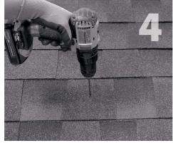
Using drill with 7/32" bit, drill pilot hole into roof and rafter, taking care to drill square to the roof. Do not use mount as a drill guide. Drill a 2" deep hole into rafter.
