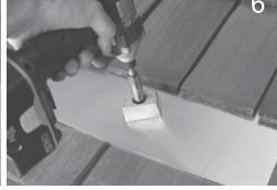
Using drill with 1/4" long bit, drill pilot hole into Clean off any saw dust, and fill hole with Seal-Slide Mount back into position. Prepare Hanger roof and rafter, taking care to drill square to the ant. roof. Do not use Mount as a drill guide.
