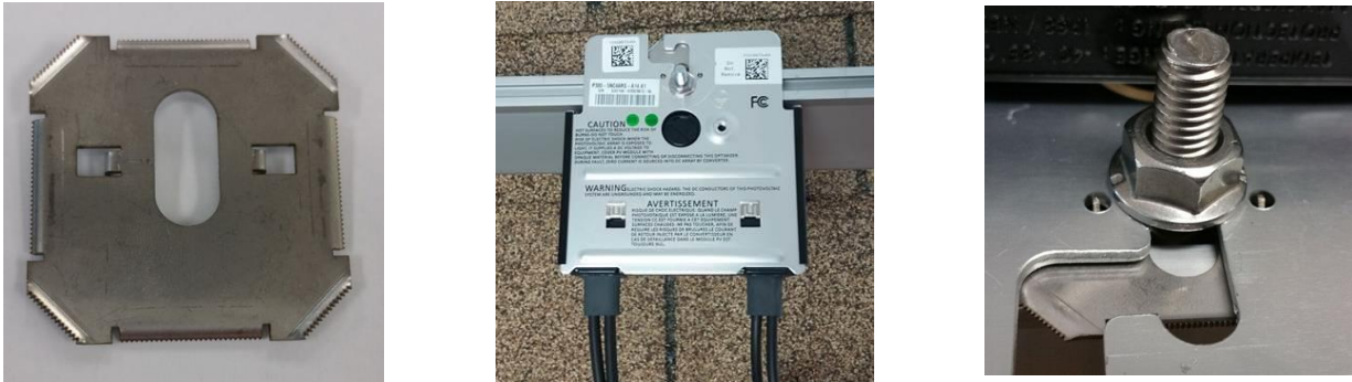
Figure 2: Grounding plate
