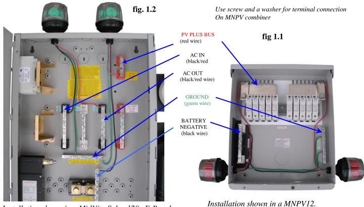
Installation shown in a MidNite Solar 120v E-Panel.
