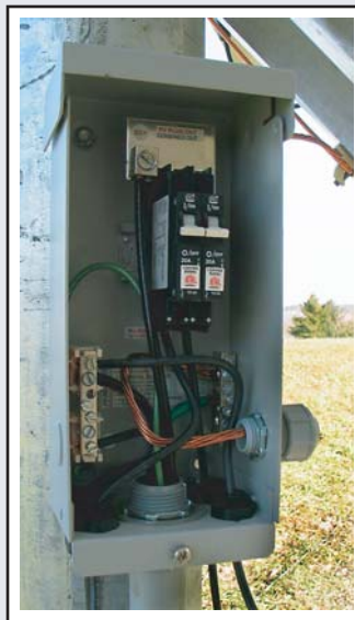
Installation photo courtesy of APRS World
